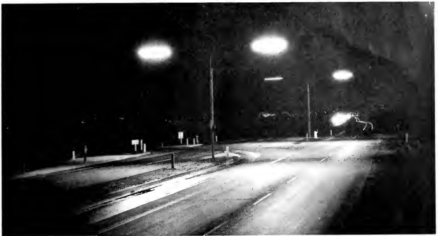
Night view on US 101 in Arcata during wet weather, showing broad band of light across intersection and its approaches provided by the new-type luminaire
